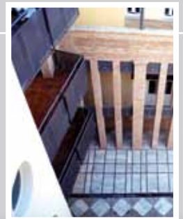
Building remodeling construction project in party walls for dwellings, commercial space, garages and warehouses on 7 Luis Montoto Avenue, Seville Promotor: Galia Grupo Inmobiliario
